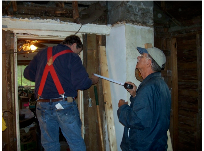
William Chewning and Rea Cooper measuring for new ceiling installation.
