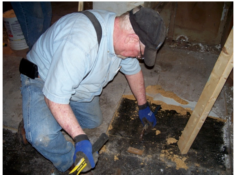
Larry Lloyd removing old flooring.
